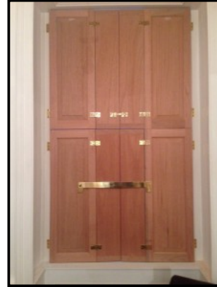
Typical split shutter set with 2ft shutter bar
